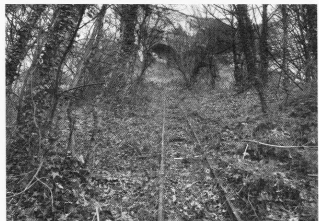
Narrow-gauge contractors rail incline used during the excavation of the tunnels at Dumpy Level. Photo by Nick Catford
